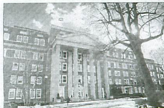
The former Medical College of Pennsylvania is being renovated. "Why build for $1 what you can only sell for 50 cents?" one investor said.
